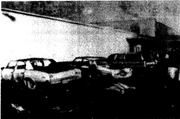
No. 5 Damage near Llewellyn Shaft
